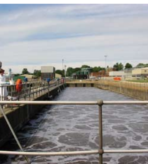
Figure 1: Example of an aeration lane within an activated sludge sewage treatment plant. Can we improve oestrogen removal here?
