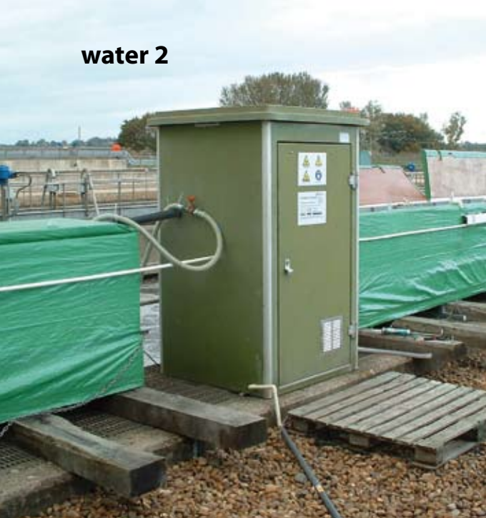
Above: Figure 4: Oestrogen removal trials in 1 m 3 flow through tanks at Northampton. Two tanks are used, one with a media filling, and the other as a control
